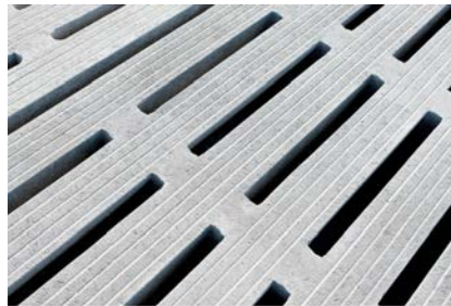
Figure 6.2 A photo showing partially slatted concrete flooring (sometimes referred to as "slotted" flooring).
