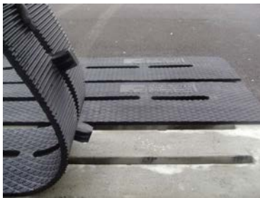
Figure 6.3 A photo showing rubber covering applied to "slatted" concrete flooring surfaces.
