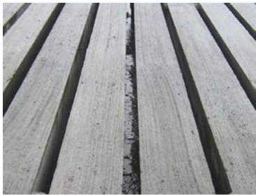
Figure 6.1 A photo showing fully slatted concrete flooring.
